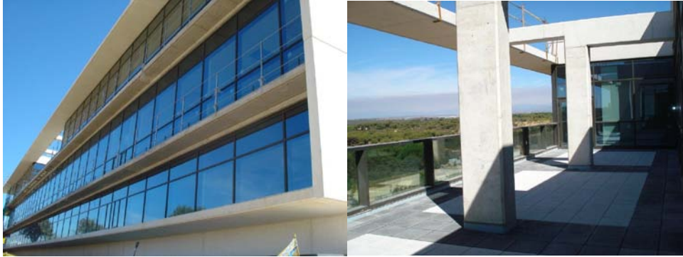
Figure: External view and the cafeteria terrace on the top floor.
