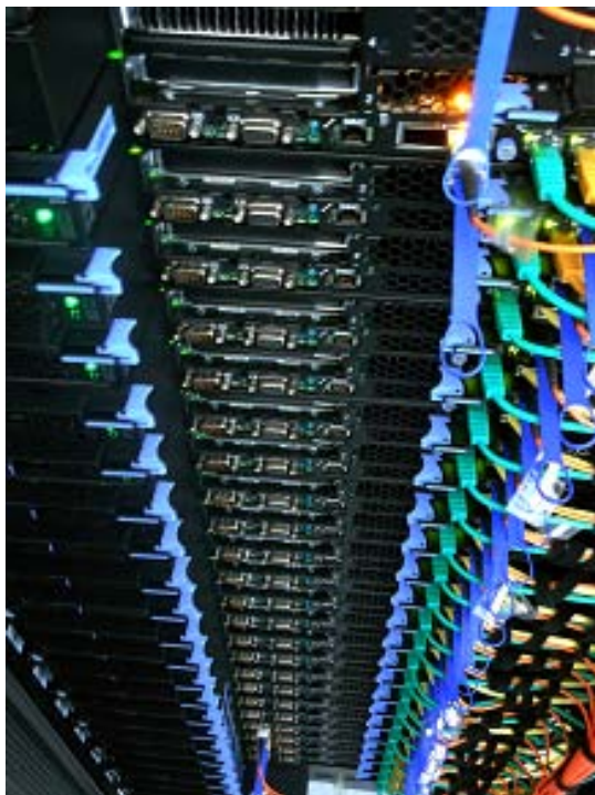
Magerit-iDataPlex in the CeSViMa
