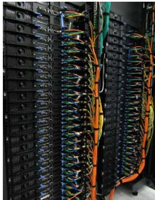
Magerit-iDataPlex in the CeSViMa
