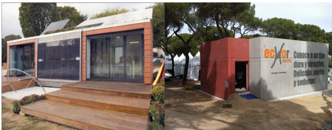
Figure 51. The UPM dwelling and the modulo donated to the UPM by ECHOR (installed in 2013)
